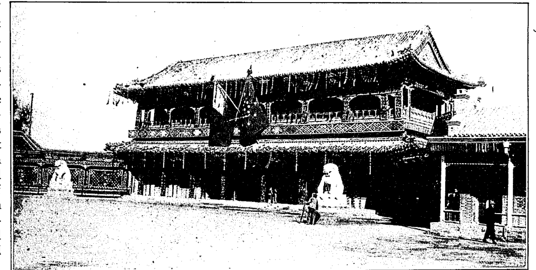
ENTRANCE TO RESIDENCE OF PRESIDENT OF CHINA
