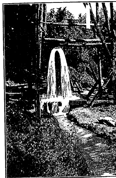
Artesian Well— One of three wells that supply the new plant with pure water at 32,000 gallons an hour.
