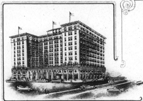
HOTEL FORT DES MOINES 400 ROOMS — 400 BATHS SERVIDOR SERVICE
