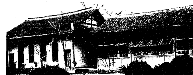
FIG. 3. Same. On the left a classroom; on the right, gymnasium; plaster walls, tile roof.
