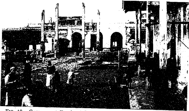
FIG. 10. Government Teachers' College for men. Main entrance. This was the inner gateway to the old Imperial City and the court between it and outer gate. Buildings on flanks used for military stables; heaps and ridges of stable waste drying in the court.
