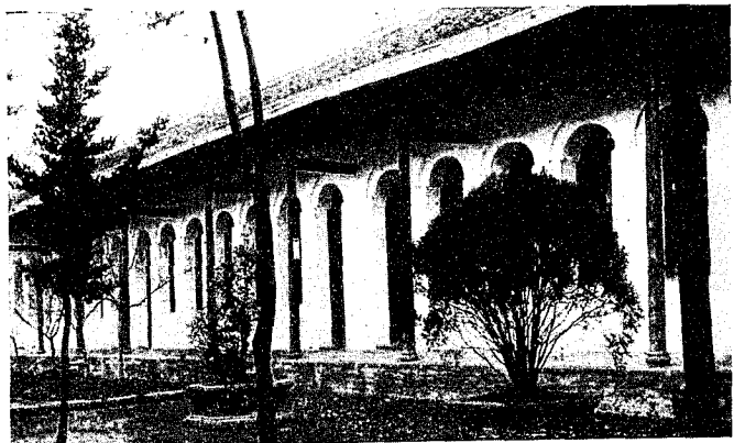
FIG. 5. Same. Court and recitation hall. A row of rooms, each entered from the covered walk along the side. No doors inside; solid walls between rooms.
