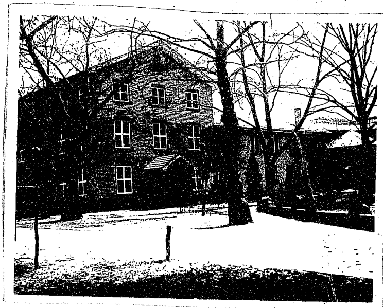
Addition to Girls' Dormitory
