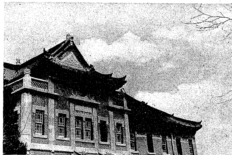
South Gable of the Administration Building
