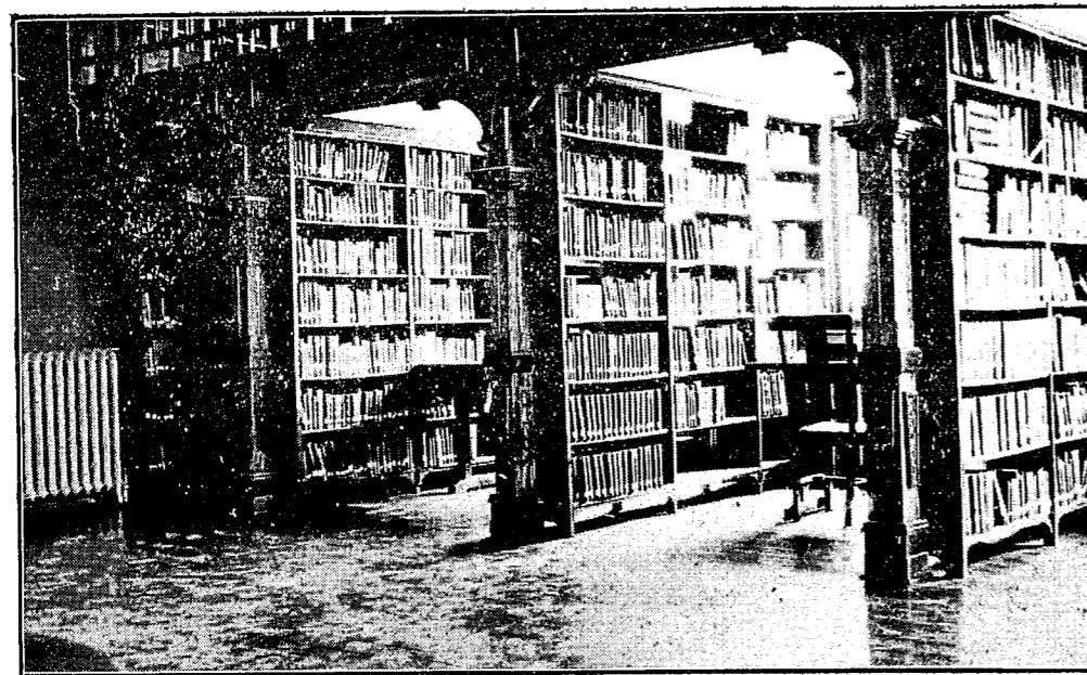
Stack Room, Library
