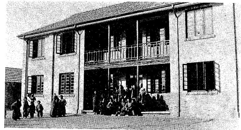
Staff and Neighbors in front of the new building.
