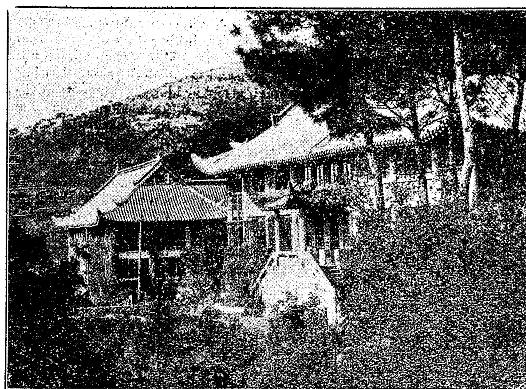
Each of the above two buildings was used as a Faculty double-residence, but they have now recently been converted into student dormitories. The third and incomplete student dormitory is behind and between these two.
