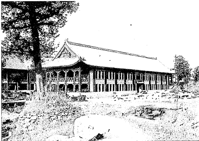
A closer view of one of the dormitories. Each dormitory houses one hundred students. Each quadrangle with additional rooms in the refectory will provide for 220 students.
