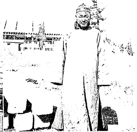
One of our foremen who is helping in the construction.
