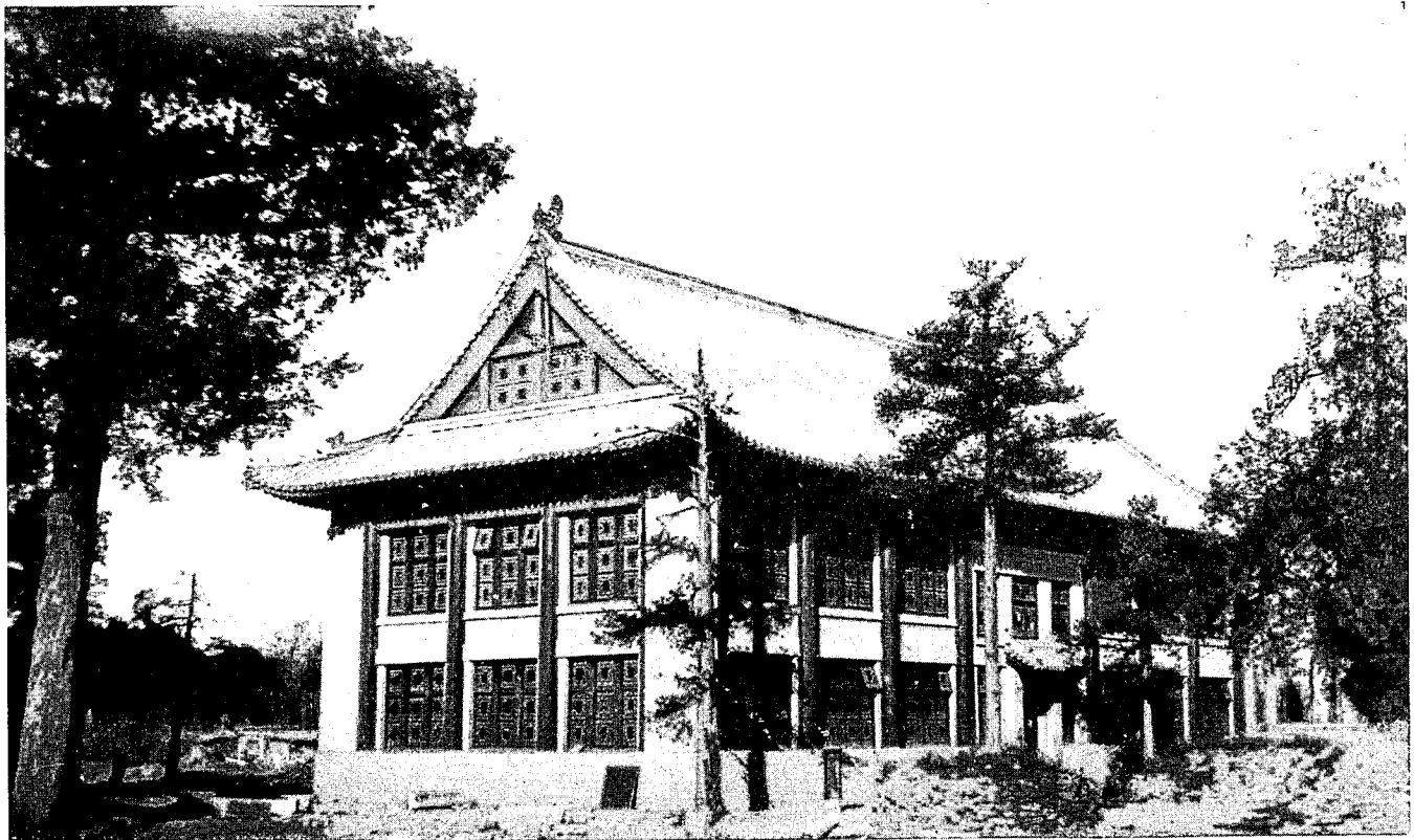
Leaded windows, red cement columns closely reproducing lacquered timber in the old palaces, highly decorated lintels, eaves, and other details—all give a rich and beautiful effect to the Yenching buildings.
