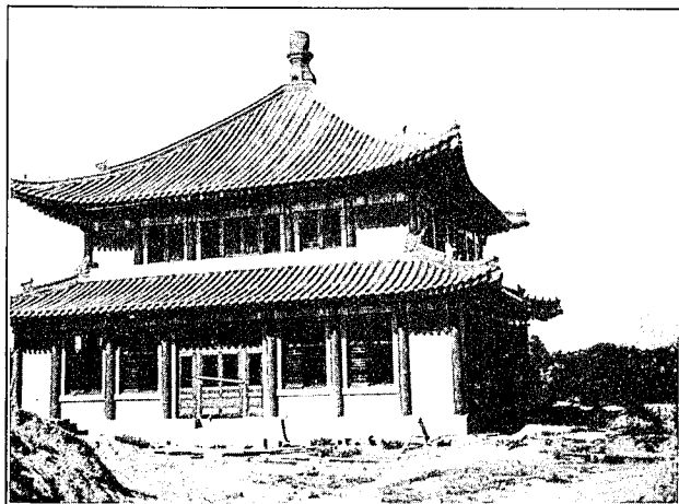
Dean's Residence (Women's College) from the northeast, Peking, September, 1924. Because of the quantities of materials stored around this building it is still impossible to get a good picture.
