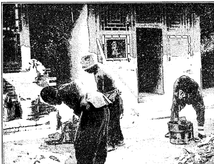
Remodelling Old Buildings for Dormitories
