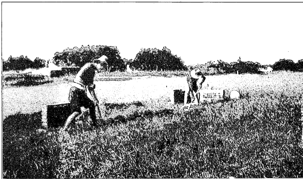
Breaking ground on the East Residence Site. Peking, August, 1924.
