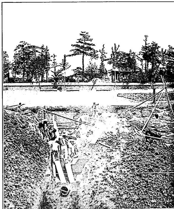
Excavation on the New Site
