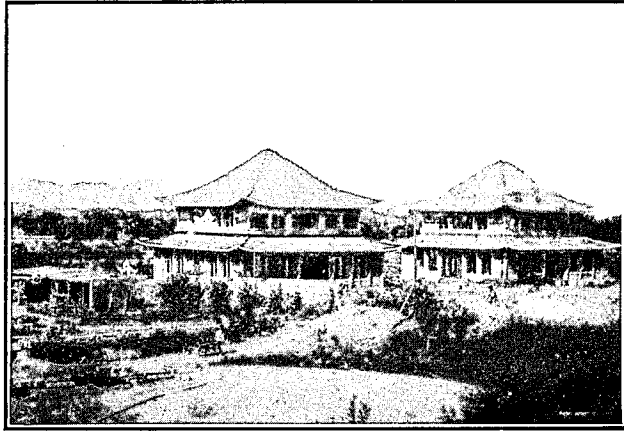
DEAN'S RESIDENCE AND ADMINISTRATION BUILDING OF THE WOMAN'S COLLEGE
