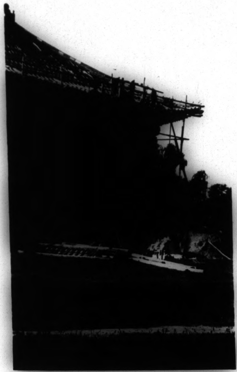
REPAIRING ROOF OF M'CBRIER HALL 1947
