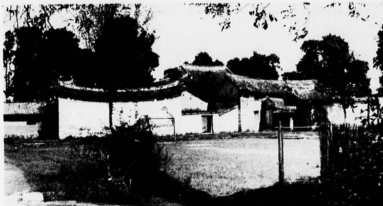
A side view of the Wartime Campus—one of several fine old temple properties now used by the College
