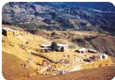
Tansen Hospital site, 1959
