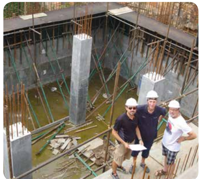
Installing the new water tank in 2015
