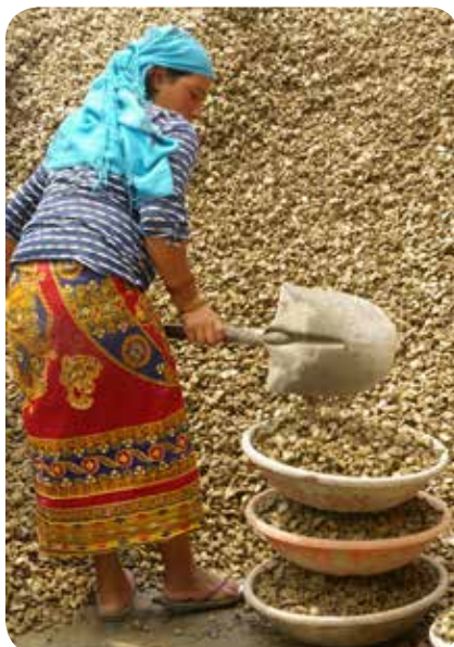
Building work at Tansen is continuous
