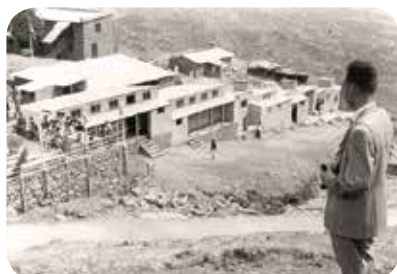
Odd Hofton at the new hospital in Tansen
